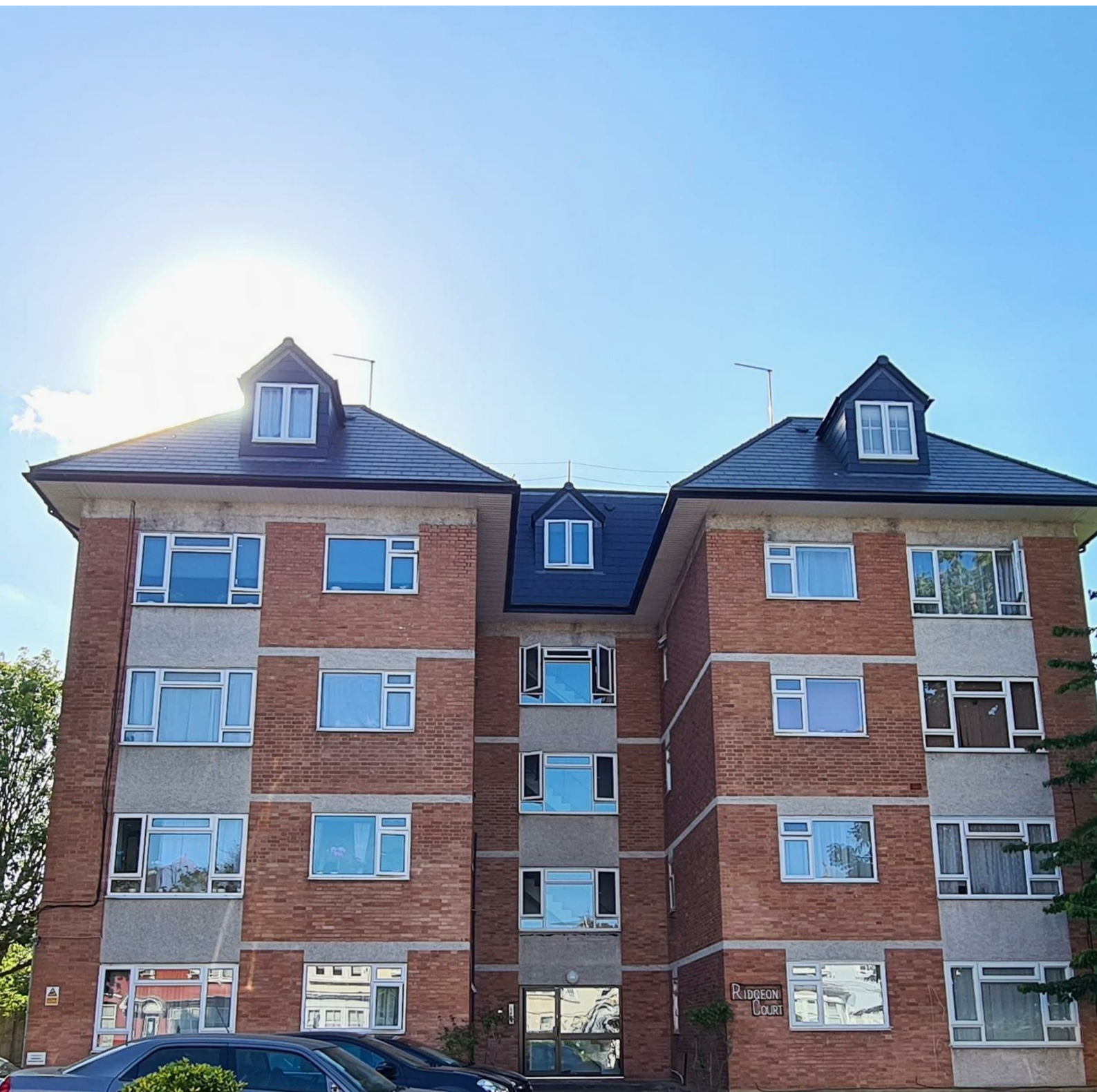
Rideon Court, Palmerston Road, Wood Green, N22
